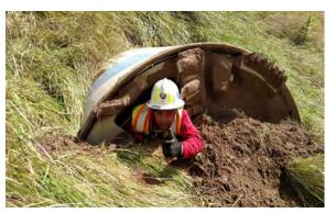
On September 11th 2017, CRS Tunnelling completed a 61m long microtunnel crossing under highway # 400 in Barrie. CRS was the tunnel subcontractor and Dufferin Construction was the General Contractor on the project. CRS installed an 1800mm RCP microtunnel pipe, manufactured by Forterra, using an Akkerman machine, under the highway to act as a
