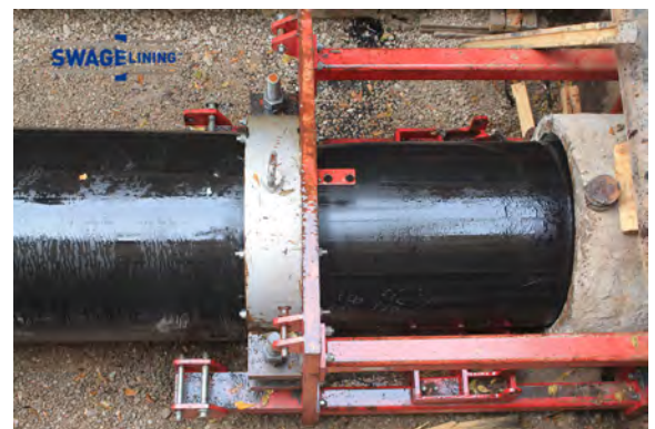
Swagelining process as HDPE is pulled through the reduction die
