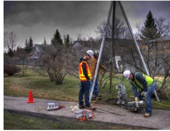
The McKenzie Feedermain, which runs through several housing communities and a provincial park, is comprised of 36-inch diameter lined cylinder pipes. The inspected sections cover a cumulative distance of 3 km, spanning a total of 438 pipes. Analysis of the data obtained during the inspection determined that 1 pipe in the feedermain was identified to have magnetic anomalies consistent with pipes that have wire break damage. In addition, 8 pipes were
