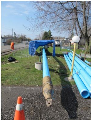
In the spring of 2011, Utilities Kingston successfully completed their very first pipe bursting project on Bath road in Kingston, Ontario. The scope of the project was to replace and upsize 720m of an existing 6" cast iron watermain that had been installed in the late 1950's. The existing pipe was showing a high failure rate and was no longer adequate to supply the volume and water pressures required in this area.
