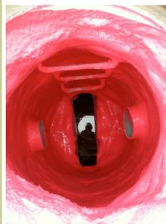
SpectraShield can be used in manholes, wet wells, head-works, grit chambers, clarifiers, aerations basins, chlorine contact chambers and large diameter pipes. Advantages of using SpectraShield include: eliminates infiltration, restores wall surfaces, prevents corrosion, environmentally friendly, trenchless applications and 100 year design life. Limitations include that the SpectraShield is only applicable to easily accessible areas and that it is difficult to apply to small diameter pipes.
