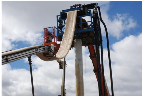
A variety of options were considered for the repair of the watermain such as: spray-on liners, slip-lining, spot repairs (e.g. internal repair sleeves), and CIPP liners. The project had added complexity, compared to traditional trenchless projects, due to the large non-standard pipe size and the watermain being suspended from a bridge
